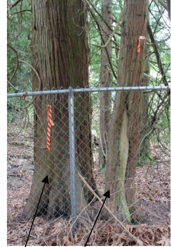
#1556 1557 Trunk and root crown decay
